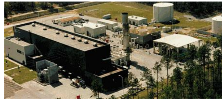
Alabama Electric Cooperative 110 MW McIntosh compressed air storage power plant
